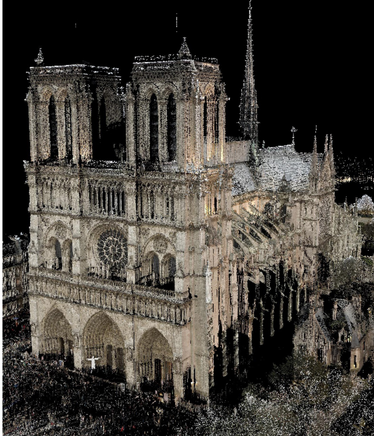
Here is an image of point cloud data of the Notre Dame. Fortunately, this cathedral had been scanned a few years prior to the fire that devastated the building. They now have the data to rebuild it exactly as it was thanks to this information.
